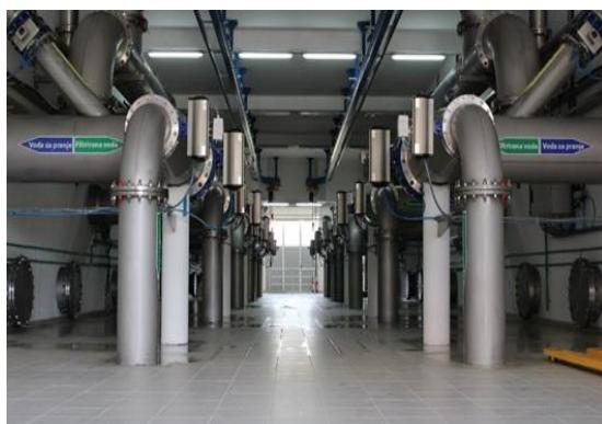
Photo 2: Tube gallery on gau filters at the new water plant (photo: Jelisaveta Dragojlović).
